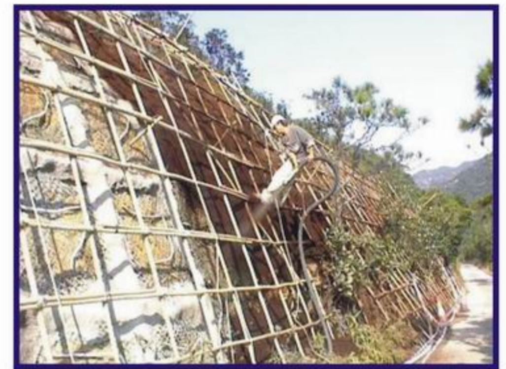
3. Spraying of Creat Bar and Fiber Soil
