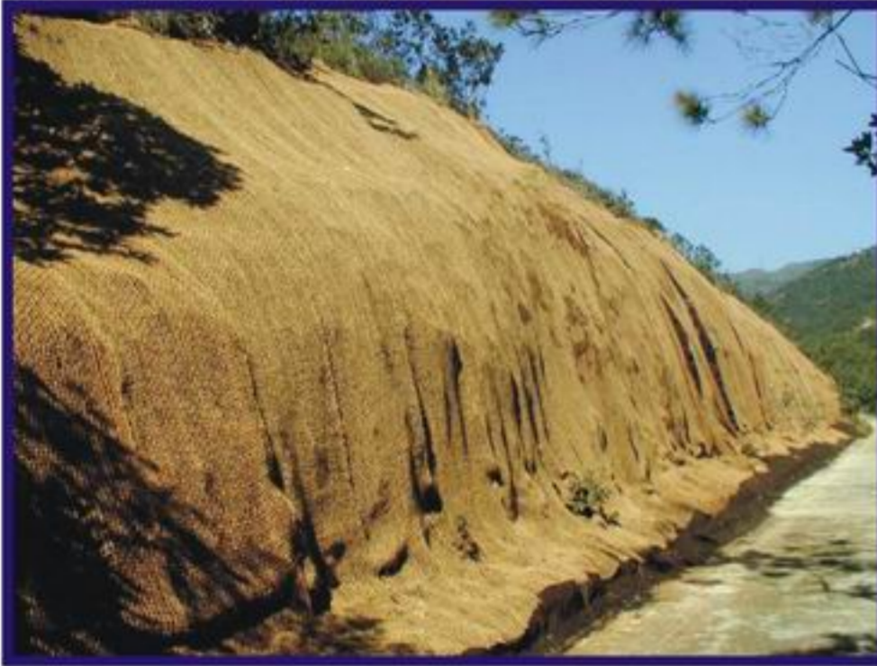
4. Laying Erosion Control Mat
