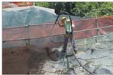
On Irregular Surface
