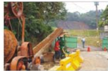
Long Distance Spraying Work
