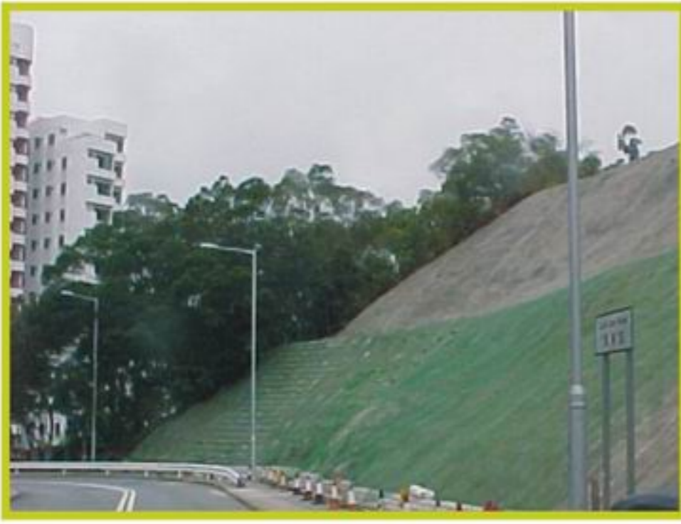
1. Fixing wire mesh by anchors
