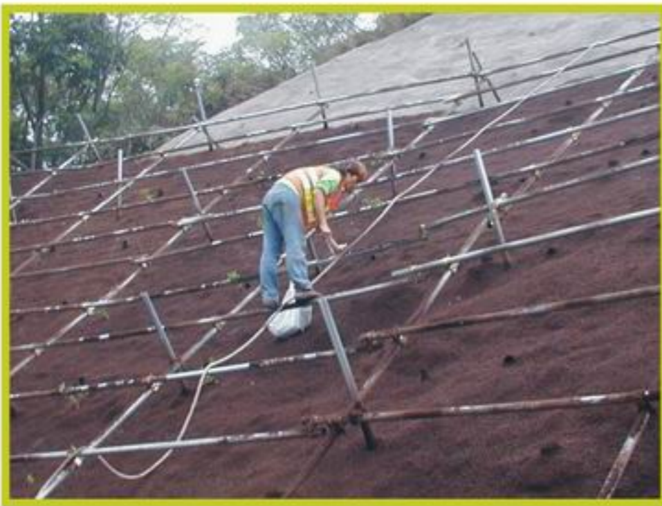
4. Installing climber sprig
