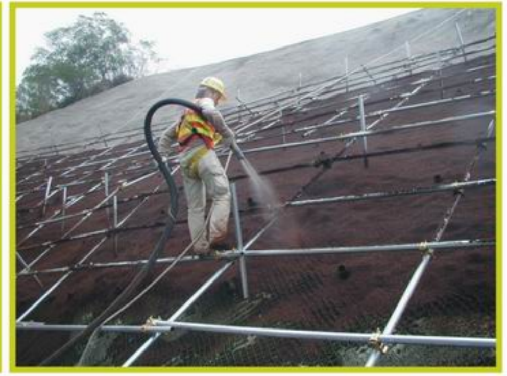
3. Spraying Fiber Soil
