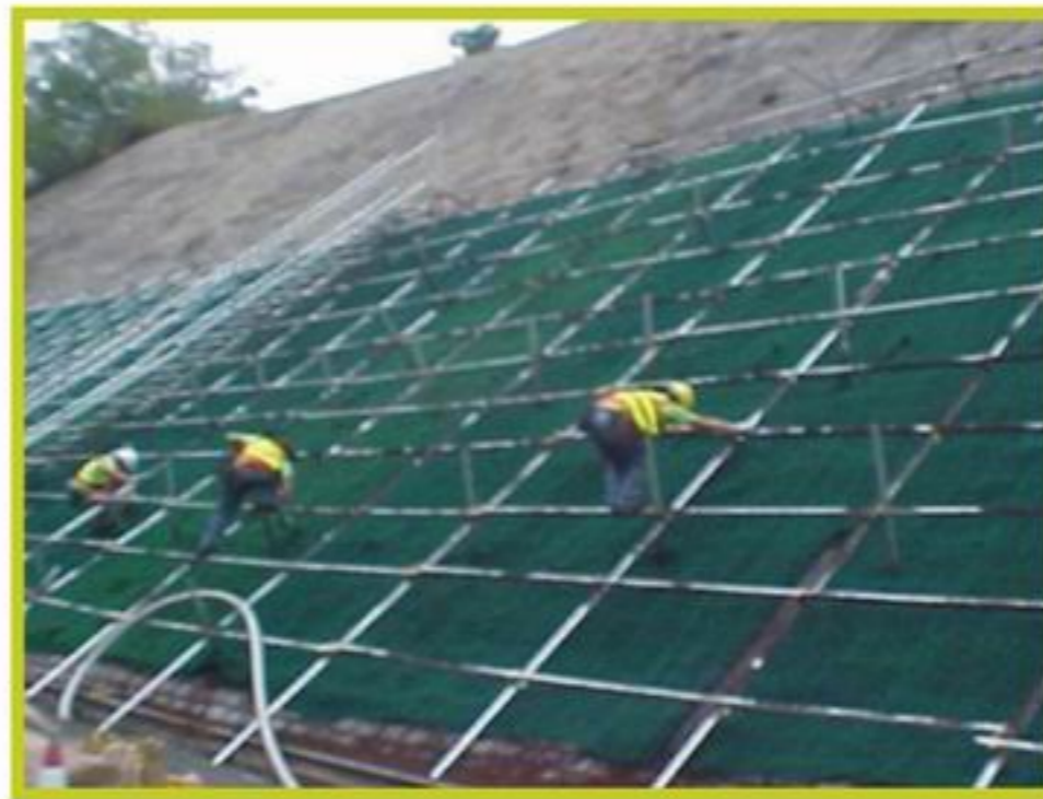
5. Laying Erosion Control Mat
