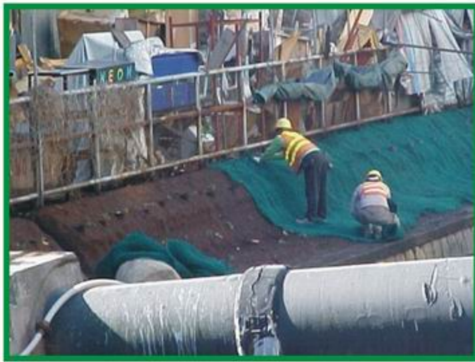
4. Fixing of Erosion Control Mat
