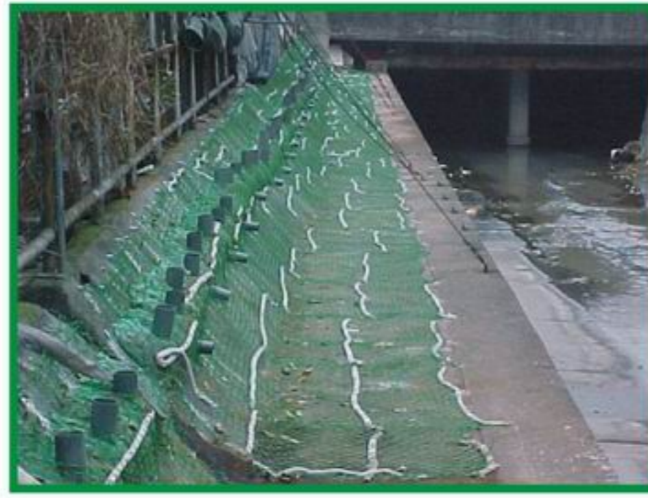
2. Fixing of Turf Reinforcement Mat & Fertilizer Strip
