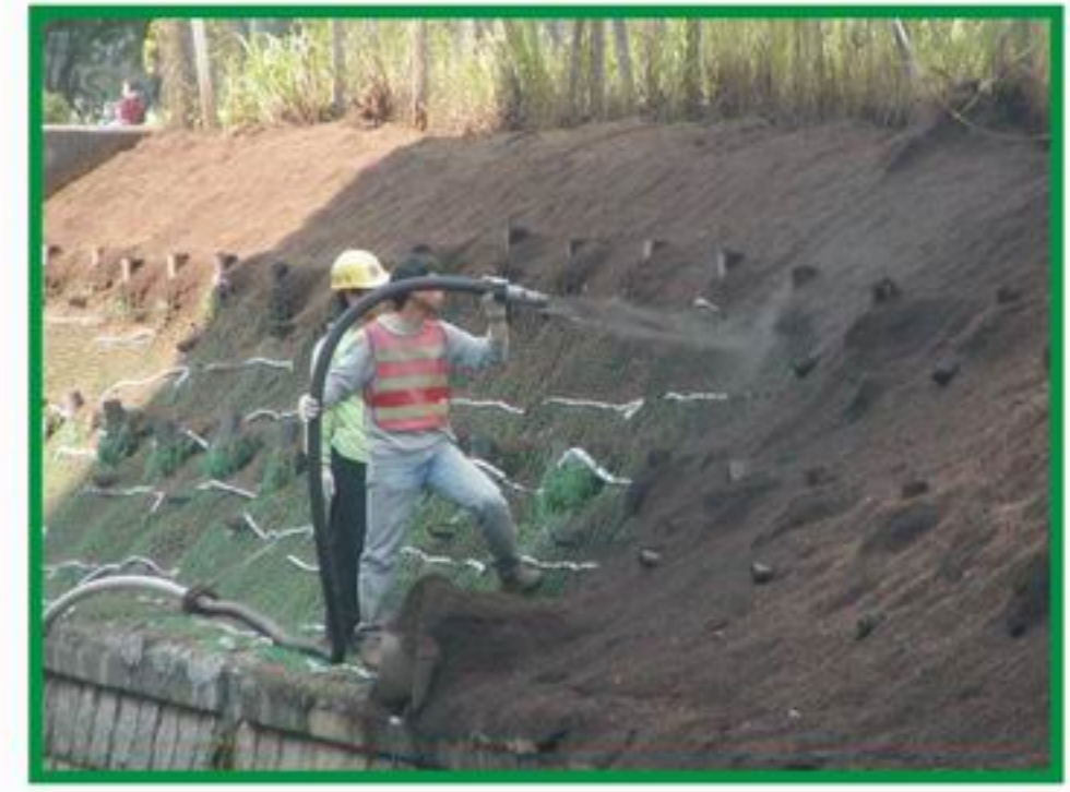
3. Spraying of Fiber Soil
