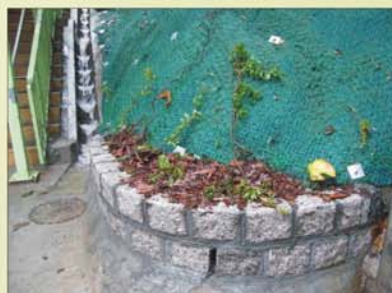
5. Back Filling of Fiber Soil with Planting
