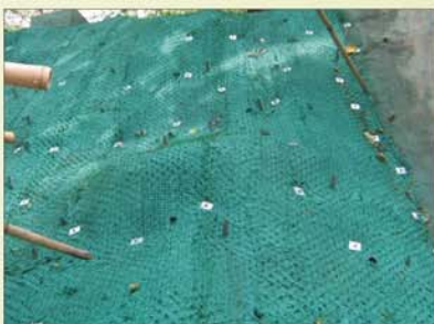
4. Installation of 3-D Rock Mesh
