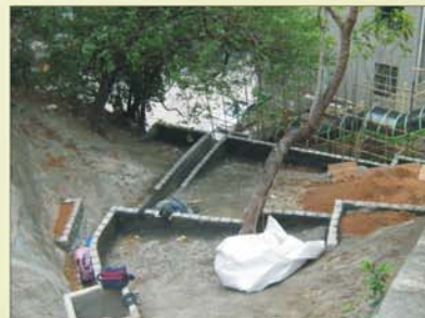
2. Installation of Toe Planter
