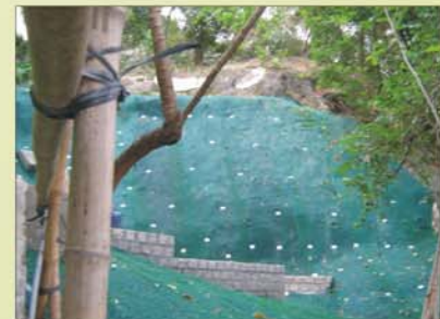
3. Installation of Geo-Net
